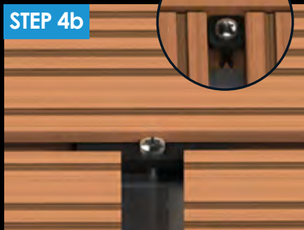
STEP 4a 4a: Half Clips can be used for different to access areas. 4b: Double Clips can be used to fix across butt joints.
